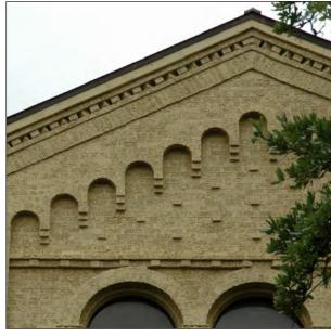
Brick articulation is encouraged as a way to create visual interest and hierarchy. Door and window lintels, sills, and floor coursing should be articulated.
