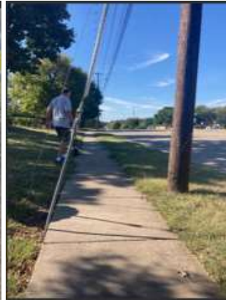
Figure 5. Poles and cables blocking pedestrians and cyclists on sidewalks
