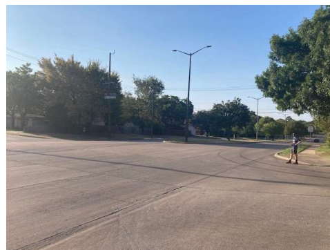
Figure 2. Crossing six lanes on S. Center Street (each lane is 12 ft wide)
