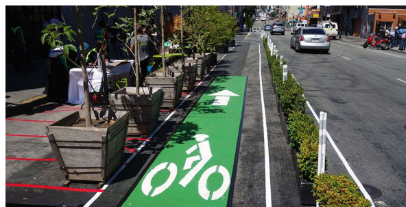
Figure 33: Pop-up Bicycle lane in San Francisco with paint, delineator posts, and planters. Source: San Francisco Bicycle Coalition
