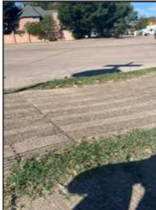
Figure 3. Overgrown grass blocking textured markings
