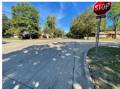
Figure 28. Lynda/Brookview intersection. This intersection can use traffic calming measures such as a roundabout.
