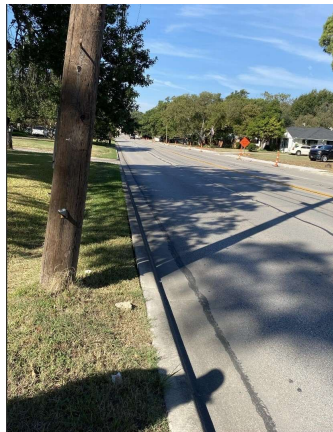
Figure 24: No sidewalk and no buffer between grass and street
