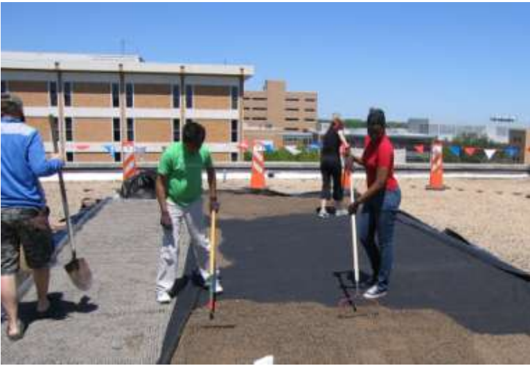
Figure 8: Growing media is placed over filter fabric
