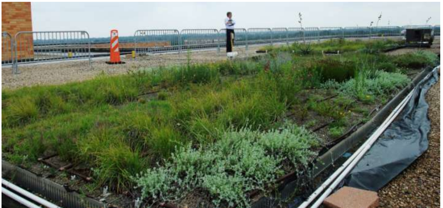
Figure 17: UTA extensive green roof test roof in the summer of 2010
