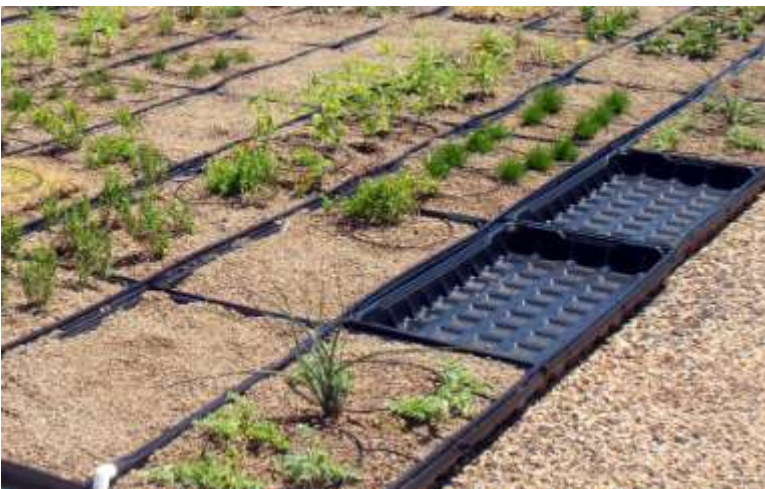
Figure 15: GreenGrid Side—partially planted out—three weeks after installation
