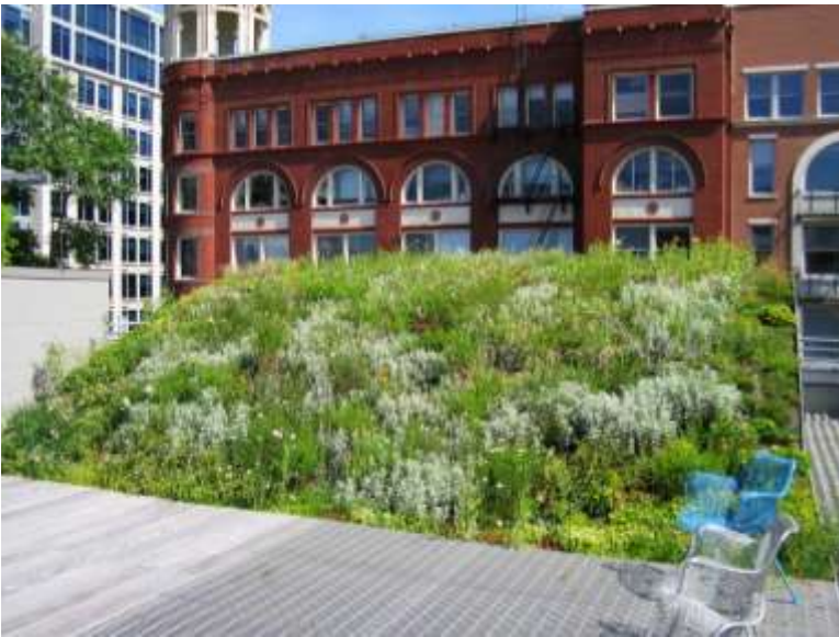
Figure 1: ASLA roof in Washington, DC showing forbs and grasses
