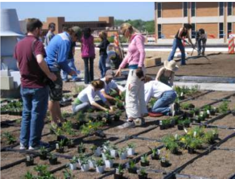
Figure 14: installing plants in the GreenGrid System
