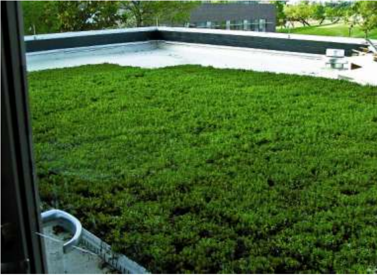
Figure 3: Sedum Roof at Northlake College in Irving, Texas soon after installation. The Sedum was pre-grown using the “Live Roof” system.
