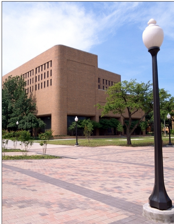
UT Arlington Thermal Energy Plant
