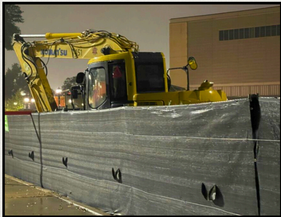
Construction on the Life Science Building | Image by Sejal Dulal
