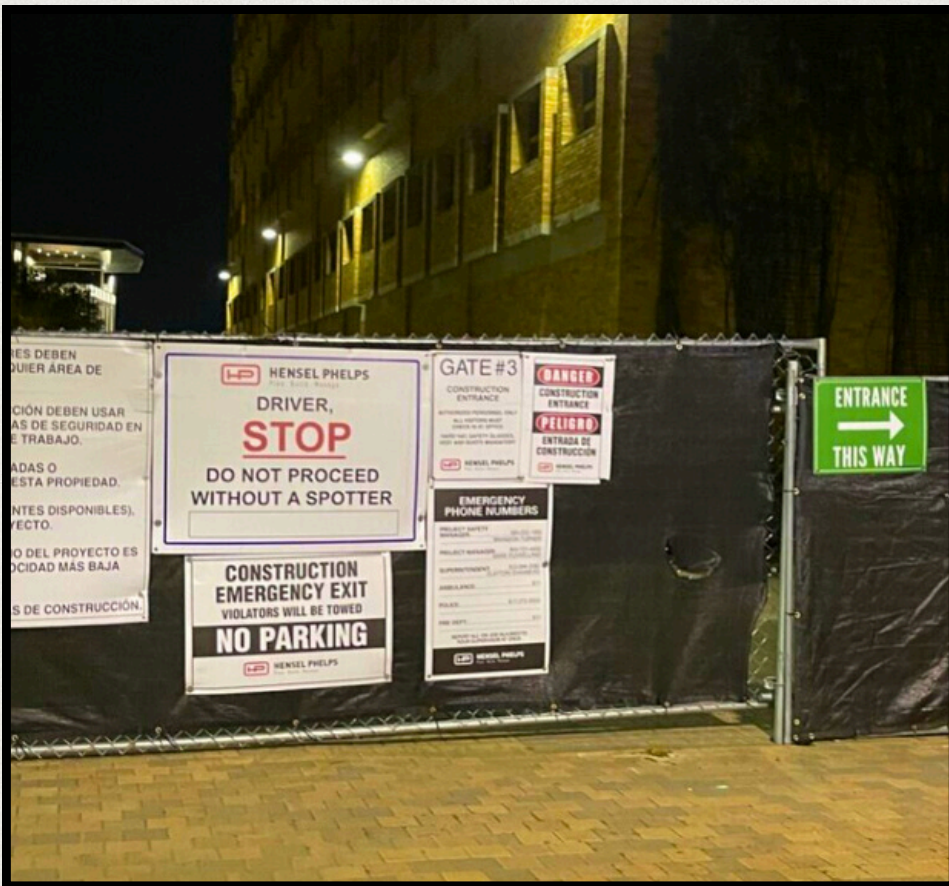
Warning Signs Around Construction Site | Image by Sejal Dulal
